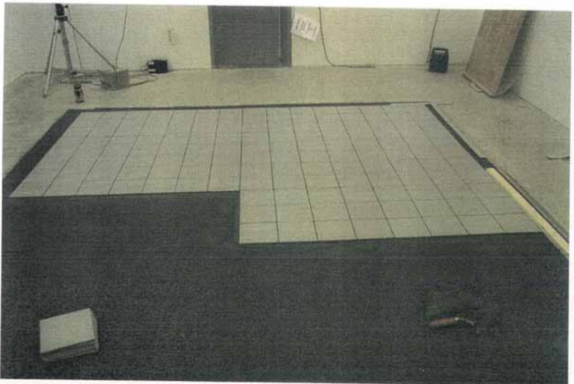
Picture 6 – The floor covering during assembly.
